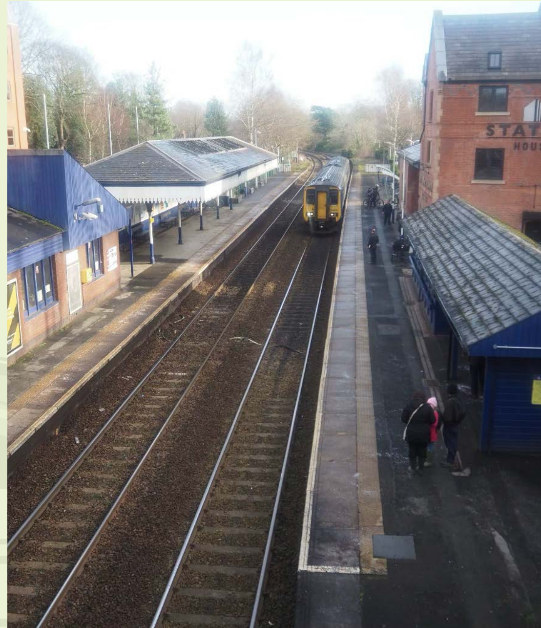
Knutsford station, Mid Cheshire line
