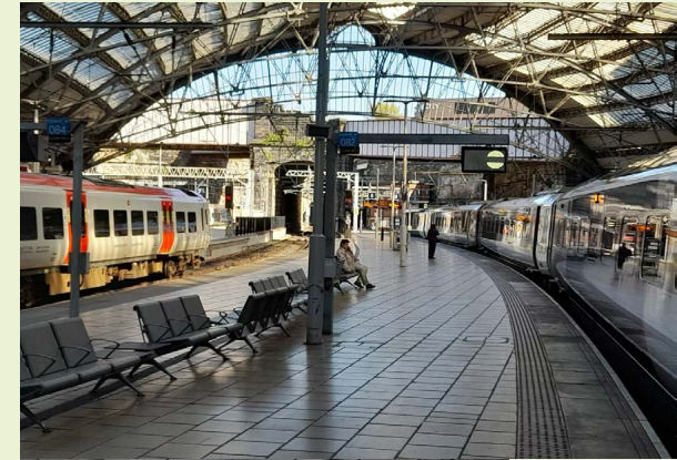
Liverpool Lime Street
