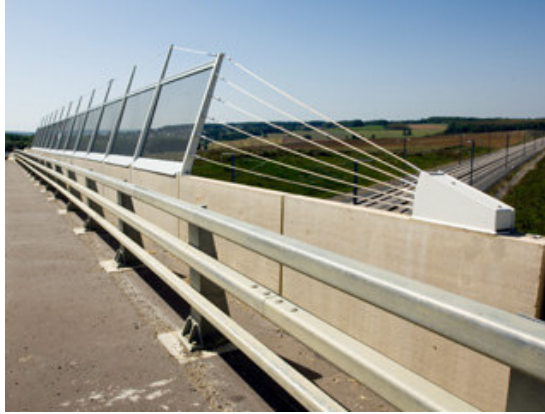
Figure 17: Added fences on road bridge
